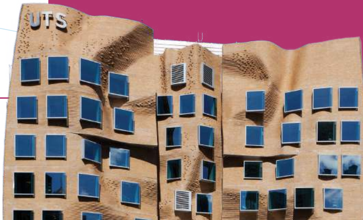
DR CHAU CHAK WING BUILDING | AUSTRALIA
